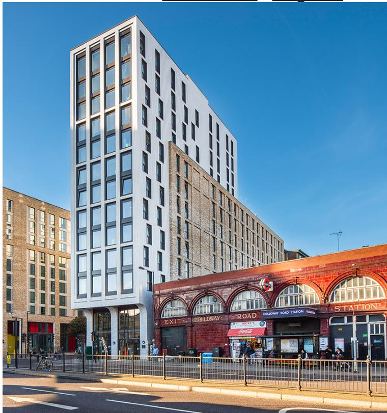
Transport for London, Tide Construction and Vision Modular Systems have completed a 12-storey, 308-module student housing scheme on top of Holloway Road Underground station, N7.
